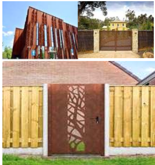
Rust Free Steel Gate & Façade Made from Corten Steel Plate/ Sheet
